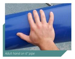
Thick pipe (3-6") is too large for many swinging movements. Its diameter makes it appealing for jumping and vaulting and can add significant rigidity to structures. At 5" or larger, pipe begins to act more like a walltop while adding visual interest and movement variety.
